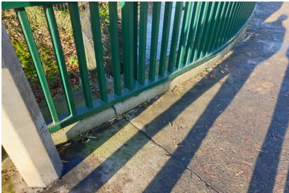
Expansion joint and railing
