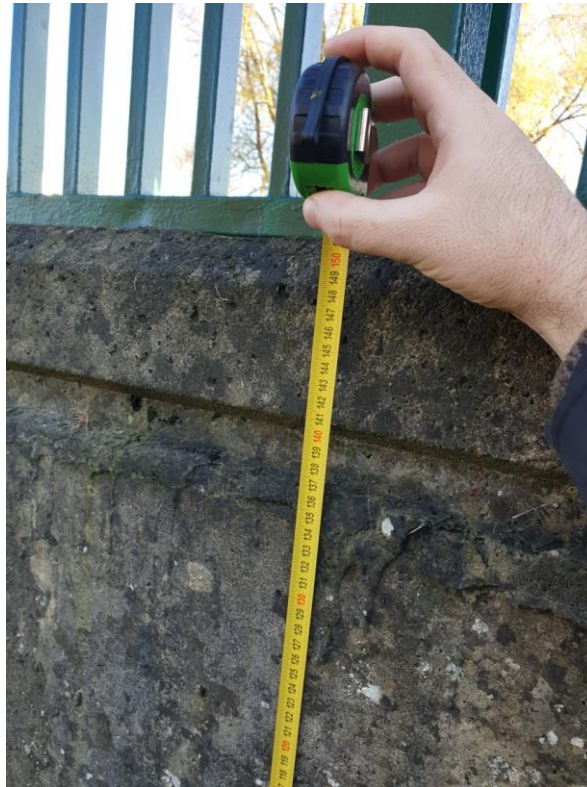
Figure 5: Measuring the depth of the slab
