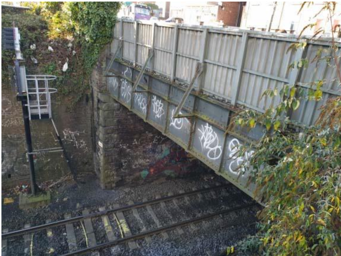
Figure 6: CBC03-02 (OBO11) Existing Parapet to be removed for bridge widening
