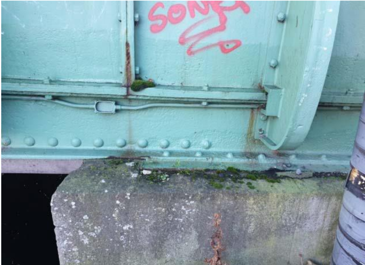
Figure 7: Cross Guns Bridge over Royal Canal - Bridge support
